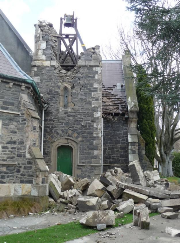
Figure 12: Collapse and vertical fracture of bell tower, St. John's Anglican Church [Photo by M. Bruneau].
