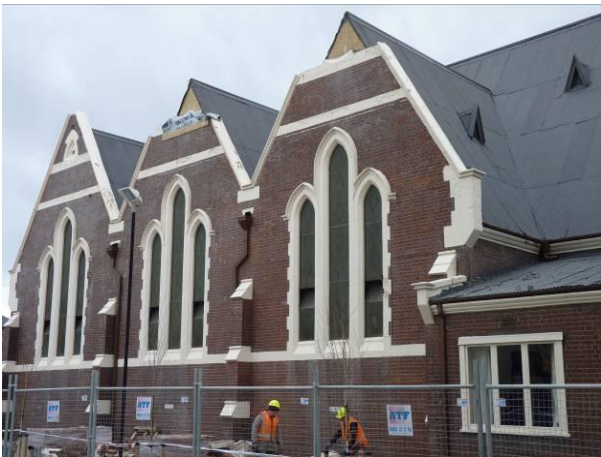
Figure 18: Damage in masonry gables and restoration, Knox Presbyterian Church [Photo by M. Anagnostopoulou].
