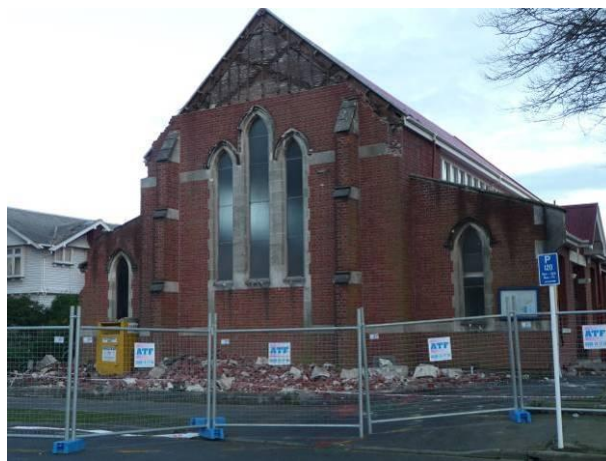
Figure 1: Out-of-plane gable failure, Christchurch Chinese Methodist Church [Photo by M. Bruneau].
