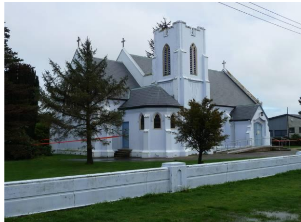
Figure 30: General view of St Joseph's Catholic Church [Photo by M. Bruneau].
