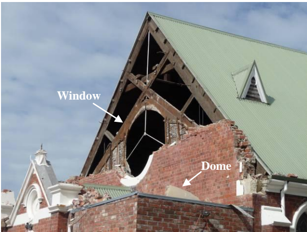
Figure 7: Failure of the façade's window and domes, St Mary and St Athanasios Coptic Orthodox Church [Photo by M. Bruneau].
