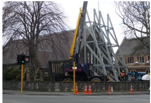
Figure 15: Reaction frame at façade's gable, St. John's Anglican Church [Photo by M. Bruneau].
