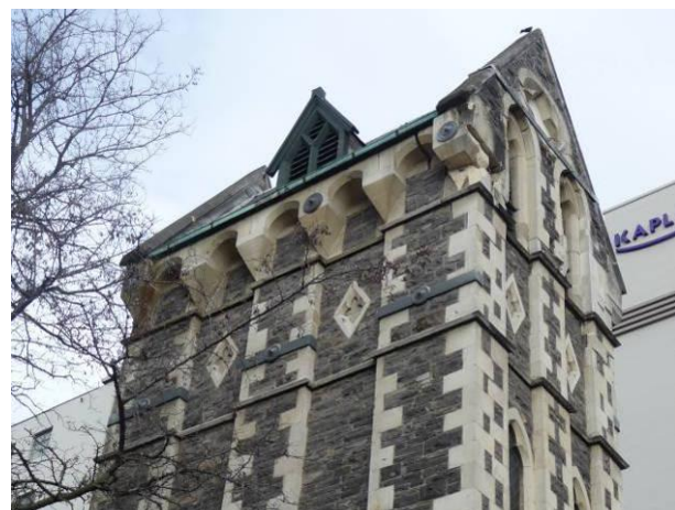
Figure 21: Anchor ties installed at building's tower, Trinity Congregational Church [Photo by M. Bruneau].
