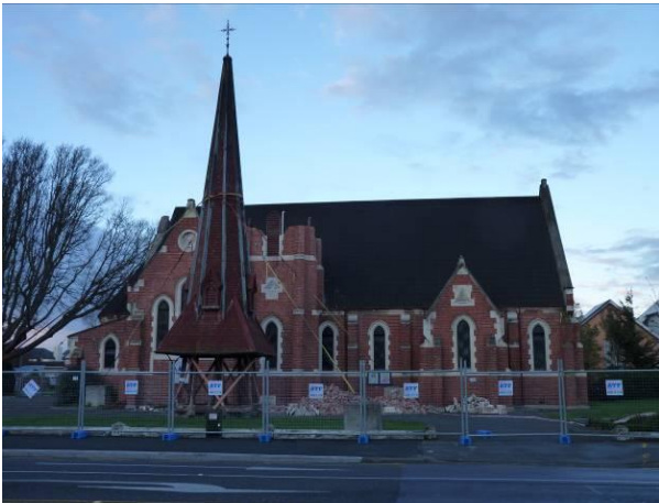
Figure 2: General view of Christchurch Chinese Methodist Church with tower and spire [Photo by M. Anagnostopoulou].
