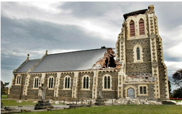
Figure 28: Collapsed tower, St John's Hororata Church (Retrieved October, 2010, from http://geoconger.wordpress.com/category/anglican-church-news/anglican-church-of-aotearoa-new-zealand-polynesia/ ).
