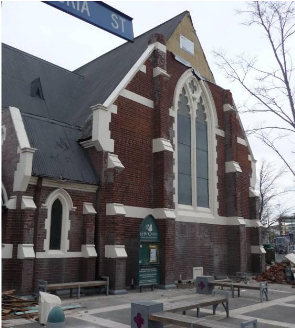
Figure 17: Gable failure, Knox Presbyterian Church [Photo by M. Bruneau].
