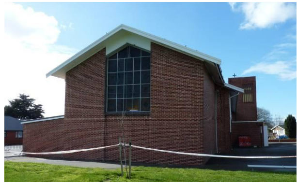
Figure 10: Ground settlement due to liquefaction, St Paul's Catholic Church [Photo by M. Anagnostopoulou].
