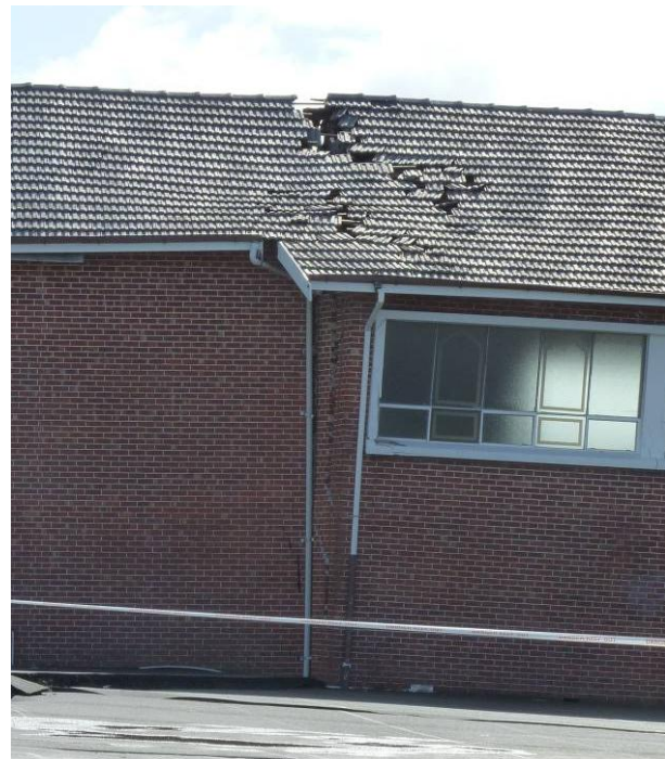
Figure 11: Gap in the roof and vertical cracking due to differential settlement, St Paul's Catholic Church [Photo by M. Anagnostopoulou].
