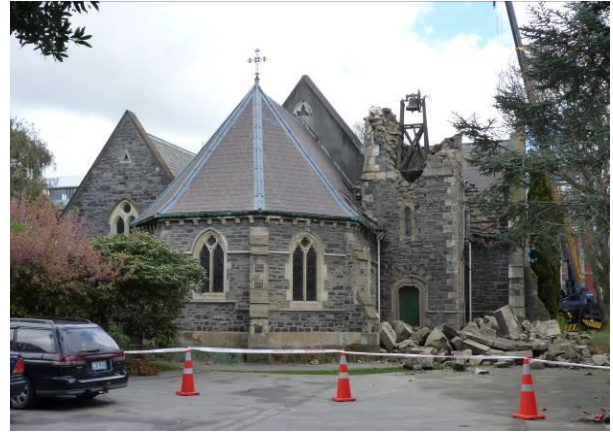
Figure 14: General view and bell tower failure, St. John's Anglican Church [Photo by M. Anagnostopoulou].
