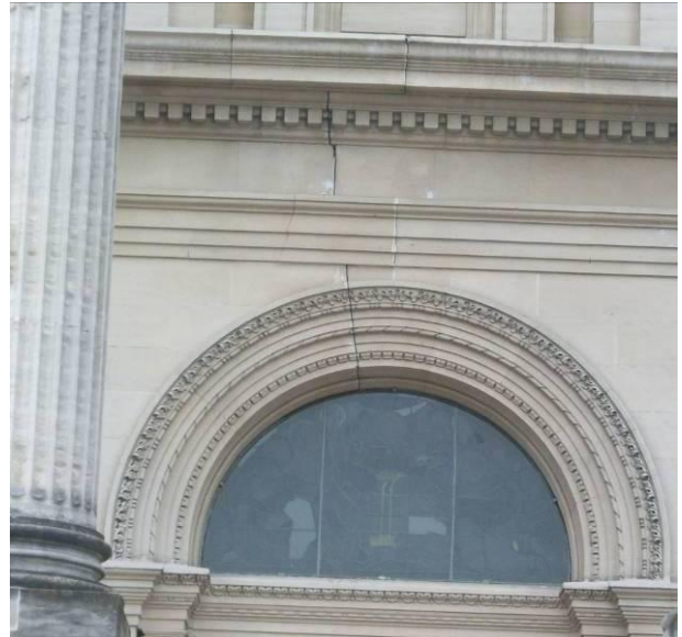
Figure 25: Cracks around keystones in the Cathedral of the Blessed Sacrament [Photo by H. Gavin].
