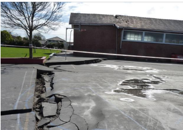
Figure 9: Liquefaction and ground deformation around St Paul's Catholic Church [Photo by M. Anagnostopoulou].
