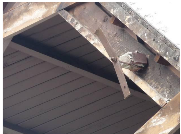
Figure 5: Characteristic type of anchor, St Mary and St Athanasios Coptic Orthodox Church [Photo by M. Bruneau].
