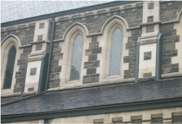
Figure 26: Steel channels along the ordinary buttresses, Christchurch Cathedral [Photo by H. Gavin].
