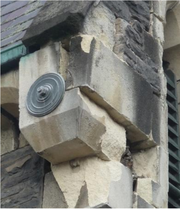
Figure 22: Damaged tower, Trinity Congregational Church [Photo by M. Bruneau].
