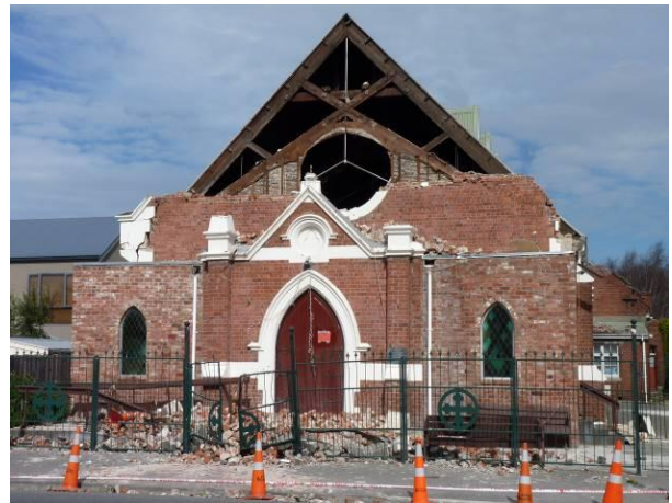
Figure 4: Front view showing significant gable failure, St Mary and St Athanasios Coptic Orthodox Church [Photo by M. Anagnostopoulou].
