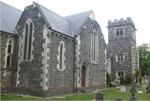
Figure 23: Fallen quire and transept parapets, St Peter's Anglican Church [Photo by H. Gavin].
