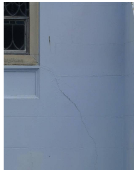
Figure 31: Cosmetic wall crack, St Joseph's Catholic Church [Photo by M. Bruneau].
