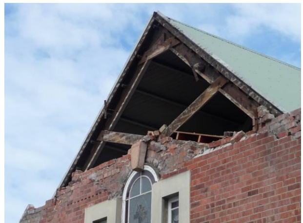
Figure 6: Masonry wall failure due to insufficient anchorage, St Mary and St Athanasios Coptic Orthodox Church [Photo by M. Bruneau].
