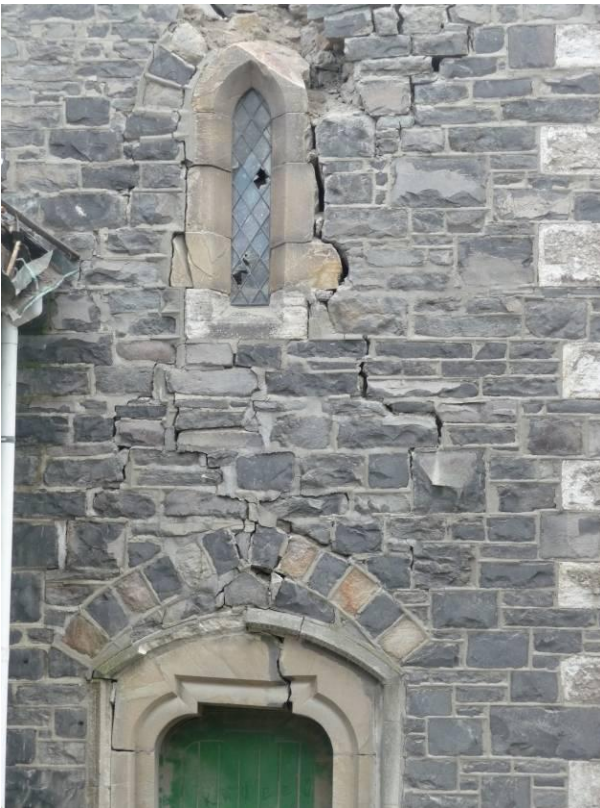
Figure 13: Vertical fracture of bell tower, St. John's Anglican Church [Photo by M. Bruneau].
