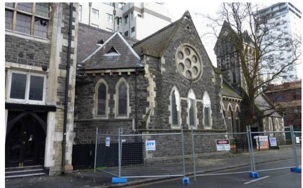
Figure 20: Side view of Trinity Congregational Church [Photo by M. Anagnostopoulou].
